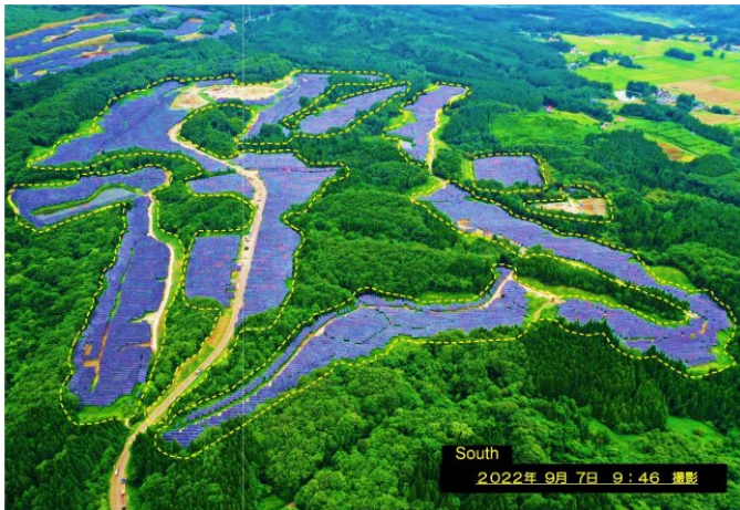
Figure 1: Onikoube's construction nears completion
